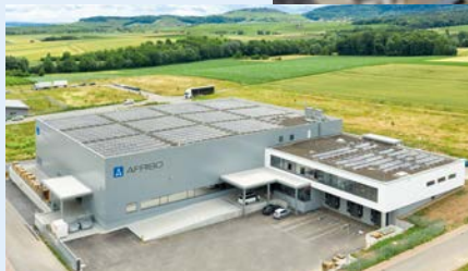
AFRISO logistics and service centre
