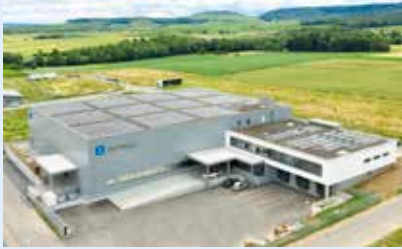
AFRISO logistics and service centre
