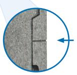
Mark at standard height of water meter (0.90–1.10 m) as a mounting aid
